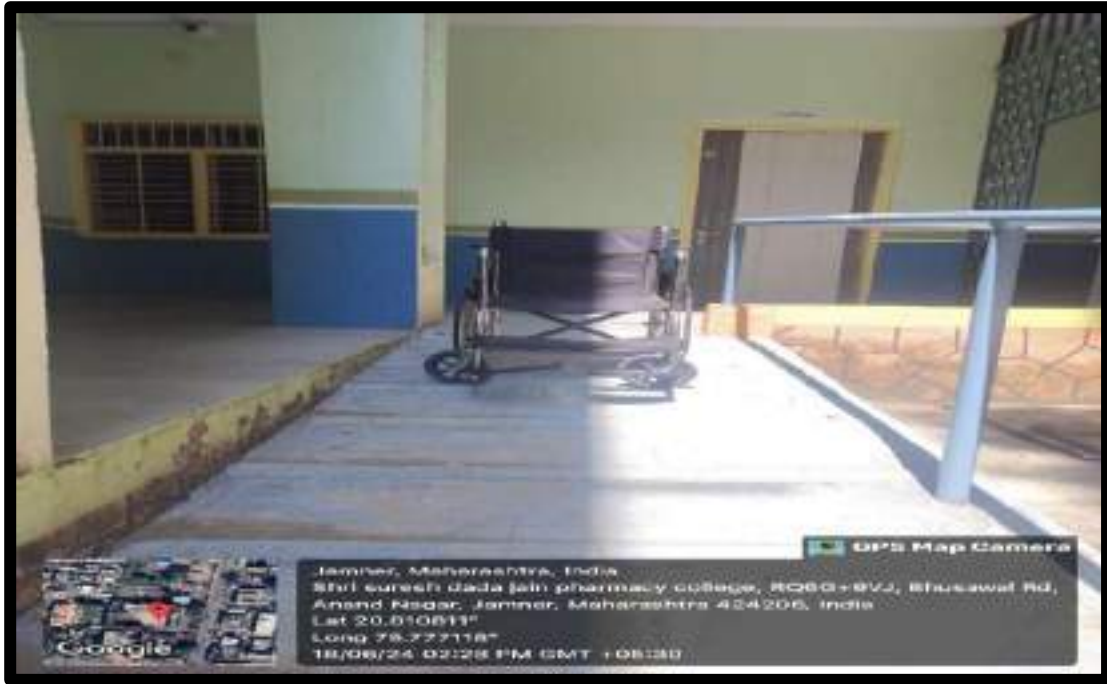
RAMP FOR PHYSICALLY DISABLED
