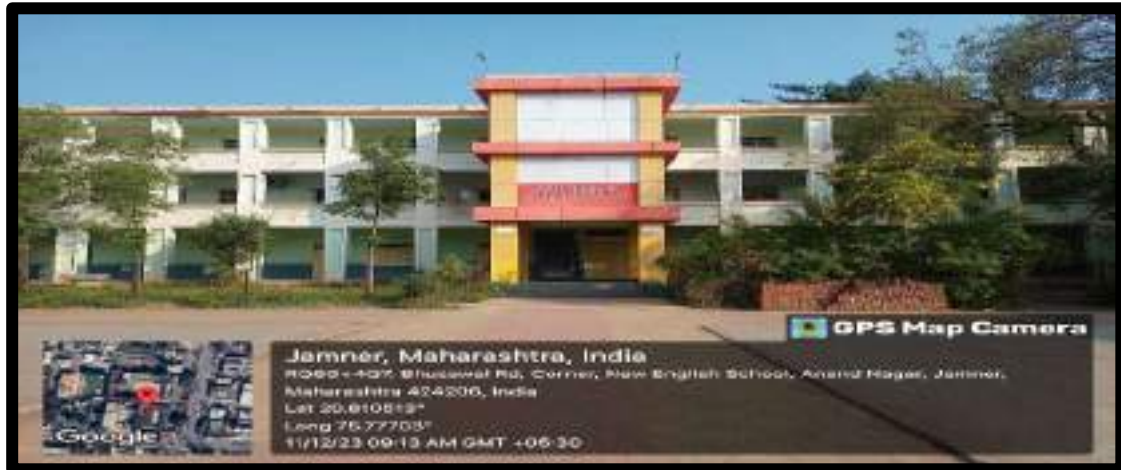
COLLEGE BUILDING ENTRANCE
