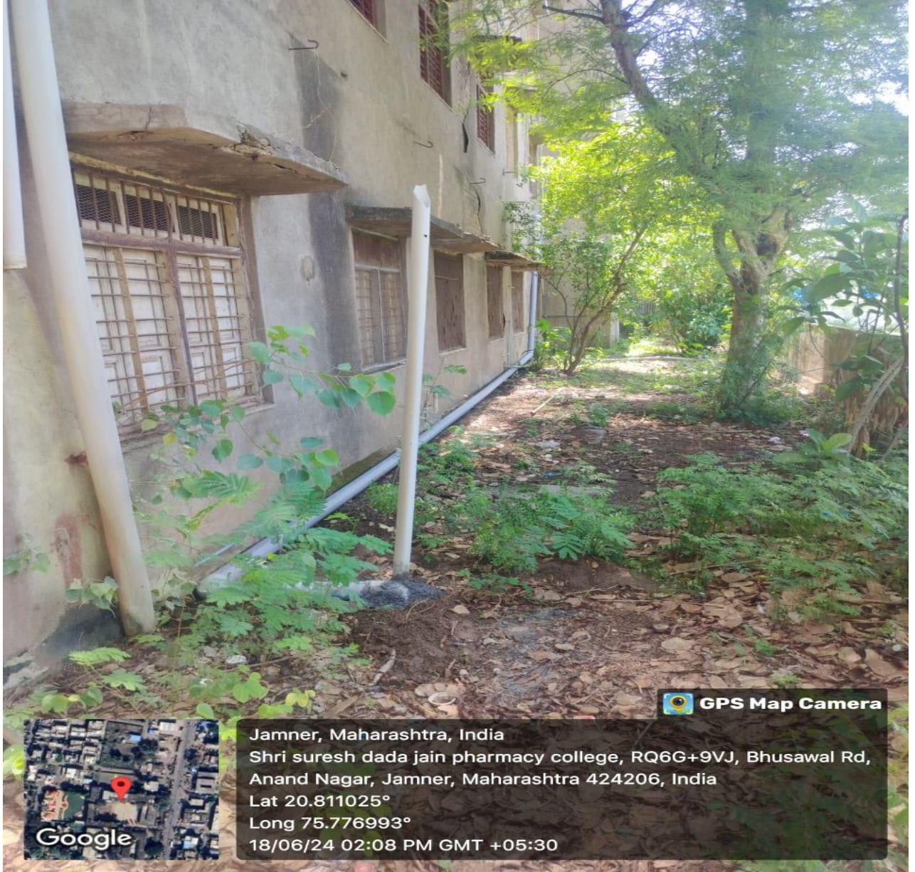
Toilet Tank Pipe
