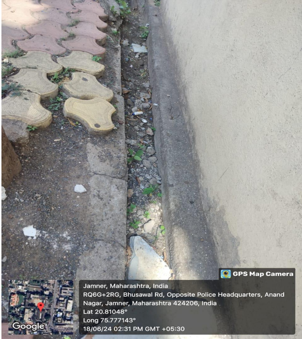
Outer Water Drainage
