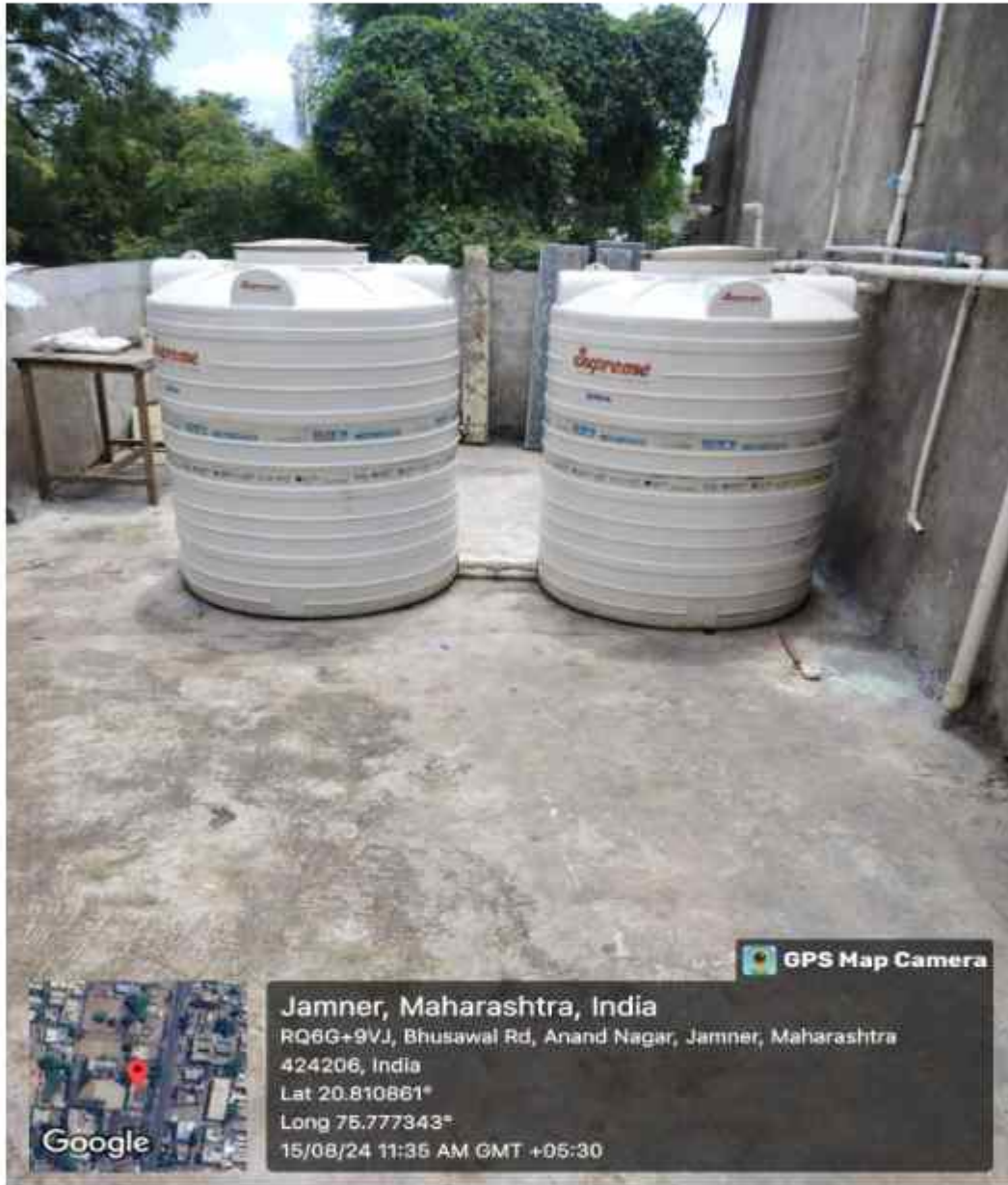
Water storage on terrace
