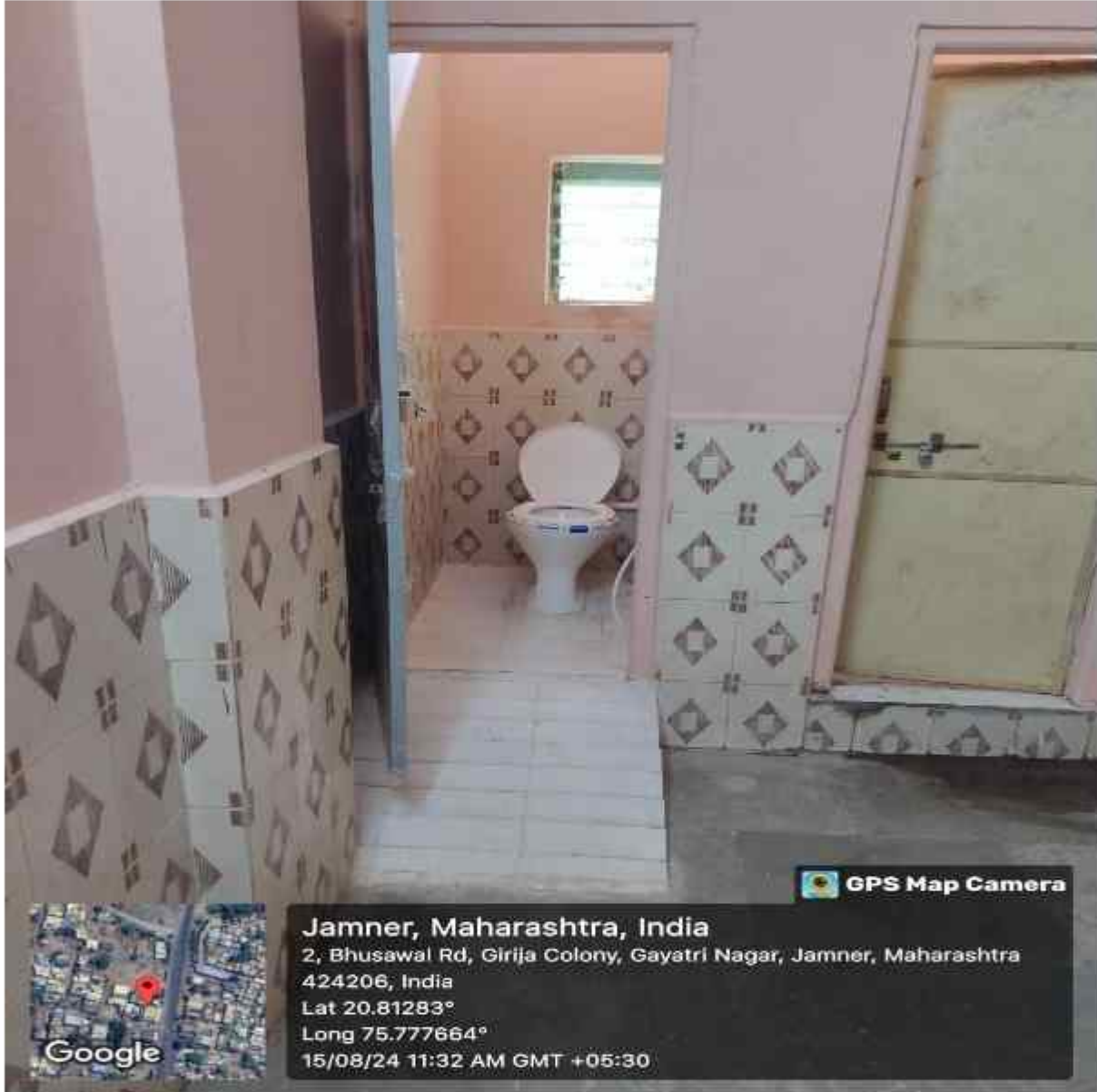
Disable –friendly Washroom
