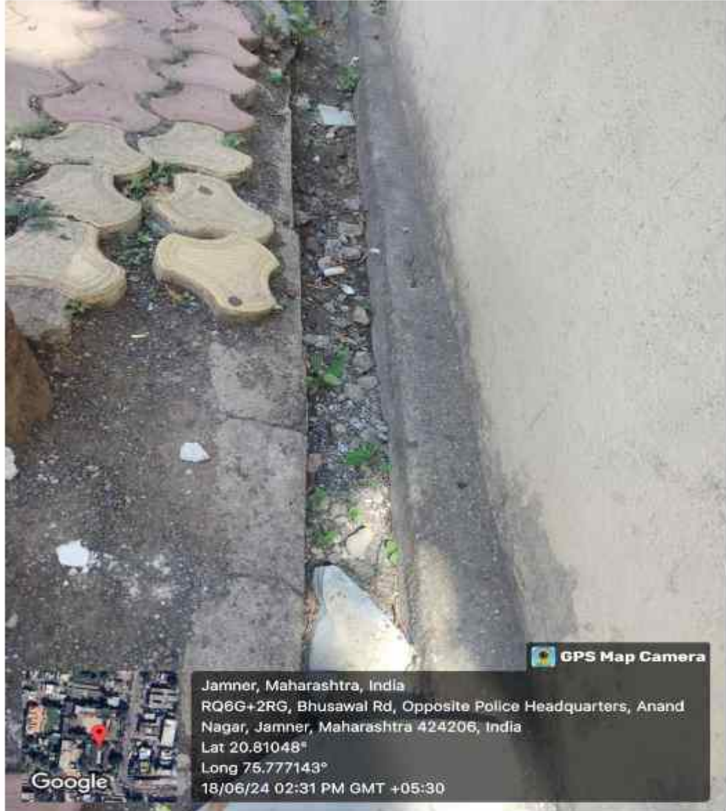
Outer Water Drainage
